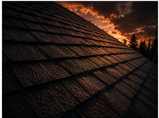
PHOTO 4 - Roof surface / shingle field example
