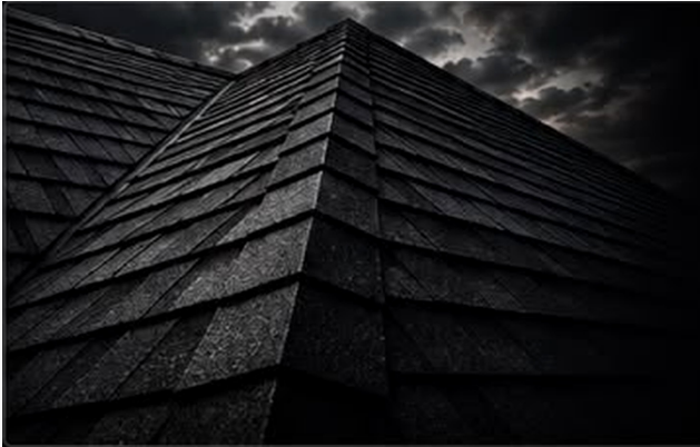
PHOTO 3 - Architectural shingle detail
